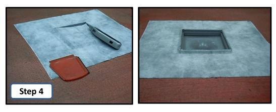
Step 4: Press the sealing sleeve with a flat object and cut on the inside a square according to the gully with a sharp knife.
