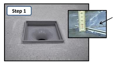
Step 1: Important!!! There shall be space for tiles and tile adhesive +2-3mm for the sealing sleeve and tanking membrane.
