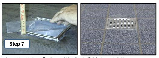
Step 7: Apply tile adhesive and the tiles to finish the installation.
